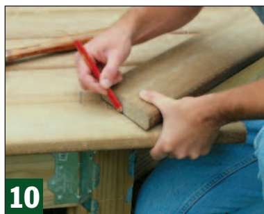
10 Mark the 22 1/2° cut off angle on the ends of the border planks. Use an adjacent plank to ensure a tight fit.
