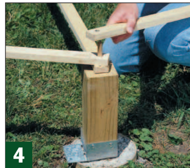
4 Use the web frame to position the posts and connectors. The frame fits on dowels centered in the top of each post.
