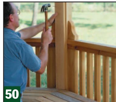
50 Nail the fascia boards (MM) to the posts inside and out. Center them to leave a uniform reveal on each side.
