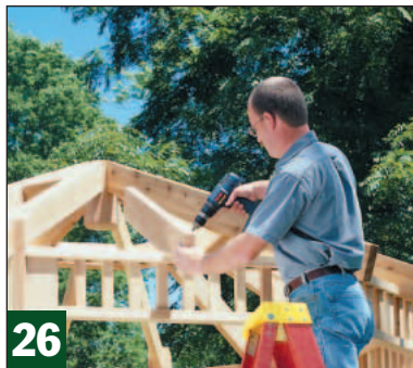
Attach the stub rafters (V) to the center of each wall panel by driving a screw through the bird's mouth notch.
