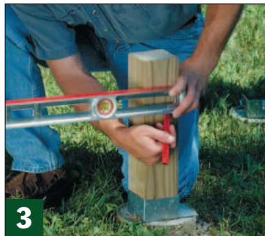
3 To mark the next post, set a level on top of the first post and mark a level line. Work from post to post.
