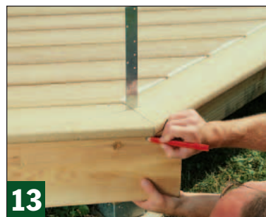
13 To determine the final length of the skirt boards, transfer the location of the miter joints from the border planks.
