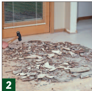
2 Demolishing the tile floor next to the kitchen exposed the subfloor so I could lay wood flooring there, as well.
