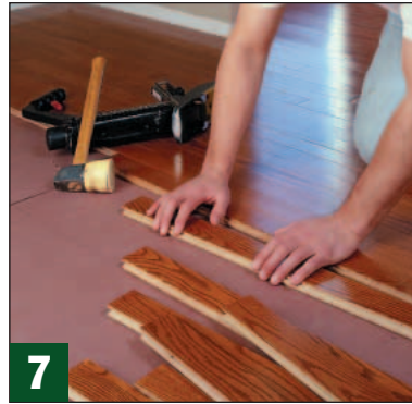
7 Racking the boards helps you select the colors, grain patterns, and lengths that blend together in the completed floor.
