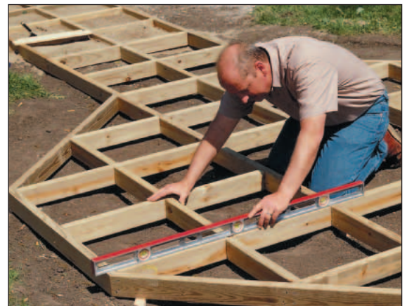
After assembling the wings (or whatever extensions you add), shim and level them to the main walkway. Then anchor the extensions with stakes and screws as before.
