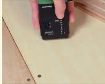
Make sure the moisture content of the underlayment is within 4 percent of the flooring before installation.
