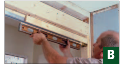
B Check that the metal track for the pocket door is level before fastening it permanently to the trimmer studs.
