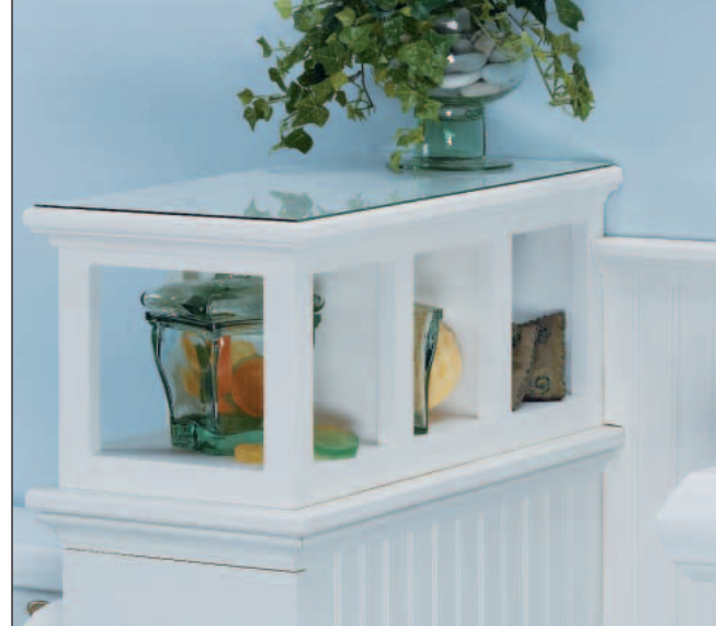
▲ The display case adds height and decoration to the partition. A piece of tempered glass protects the case cap from scratches and dents.
