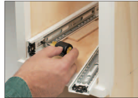
▲ Use a piece of scrap to position both slides at the same height in the cabinet.
