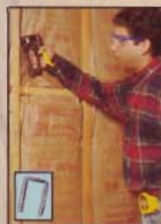
Install Insulation
