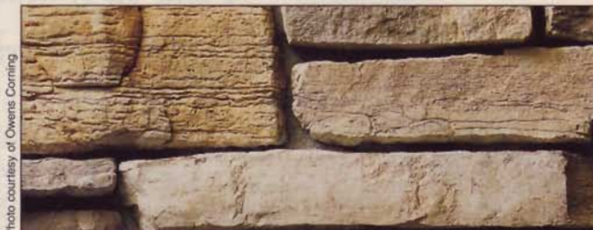
▲ Dimensional stone with grout joints.
