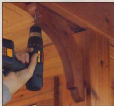
▲ The curved brackets that form a transition between posts and beams are installed with 3" deck screws.
