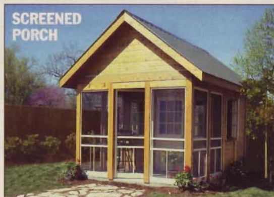
▲ To convert the front half of the building to a screened porch, simply install store-bought screen panels.
