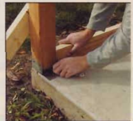
▲ To accurately determine the final location of the posts, use a board as a spacer. Then tighten the stand-offs, fold up the "flap" and fasten it with screws.
