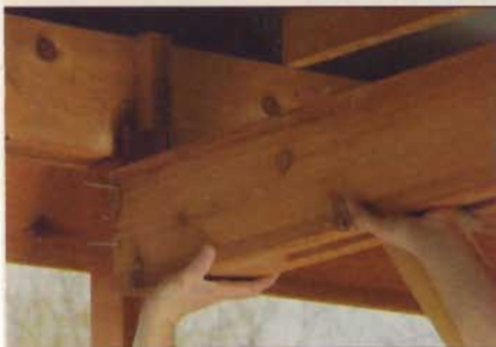
▲ All that's needed to install the interior beam is to fit it over a mounting cleat and fasten it with screws.
