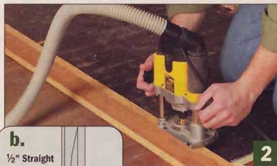
▲ Using a straightedge to guide the router, cut a rabbet in the floor. A shallow cut keeps the bit safely above any nails.
