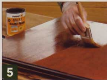
▲ To produce a soft, warm tone and restore the vivid color, brush on three coats of amber shellac.
