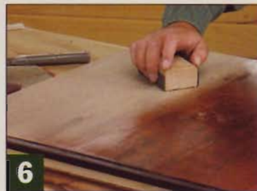
▲ Let the shellac dry, then lightly sand the entire surface smooth with 320-grit sandpaper between coats.
