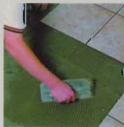
▲ A bed of mortar goes under the mat and another over it before installing the tile.
