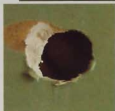
▲ The EZ Drywall Repair Kit makes it simple to fill a "door ding" (left) so the hole can be patched with drywall compound (above).
