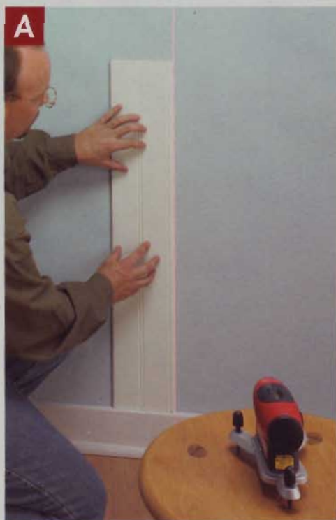
▲ Using the surface-mount base, which has three adjustable feet for leveling, turns anything from this ordinary stool to a stack of books into a makeshift tripod.
