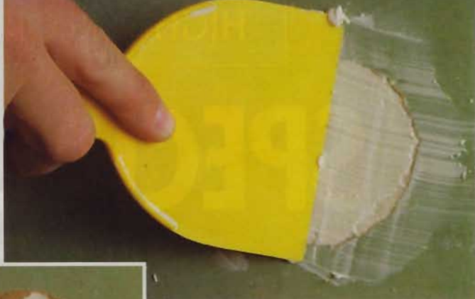
▲ The EZ Drywall Repair Kit makes it simple to fill a "door ding" (left) so the hole can be patched with drywall compound (above).
