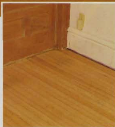
▲ After a thorough sanding, this dining room floor, originally installed in 1910, was ready for a finish (see page 76).
