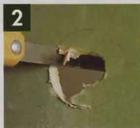
▲ The EZ Drywall Repair Kit makes it simple to fill a "door ding" (left) so the hole can be patched with drywall compound (above).
