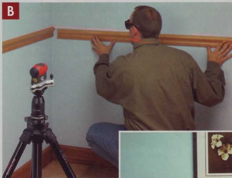
▲ A special base adapts the laser to a camera tripod. Or you can attach the laser to the wall with a wall-mount base (right).
