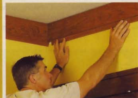
◀ After laying out the location of the beams, nail the trim boards around the perimeter. Then install a small molding underneath ( Inset Photo ).
