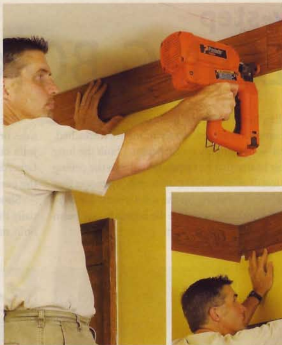
◀ After laying out the location of the beams, nail the trim boards around the perimeter. Then install a small molding underneath ( Inset Photo ).
