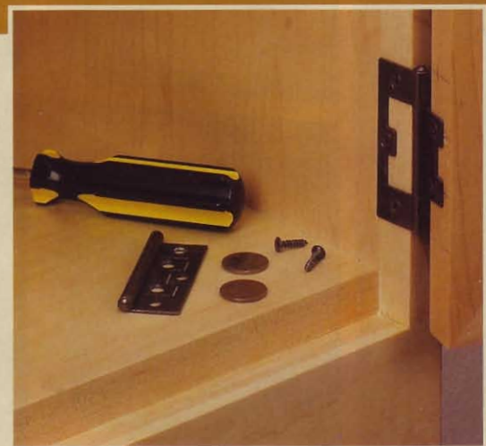
▲ No-mortise hinges make mounting the doors quick and easy. I used pennies as spacers to create an even gap around the door.
