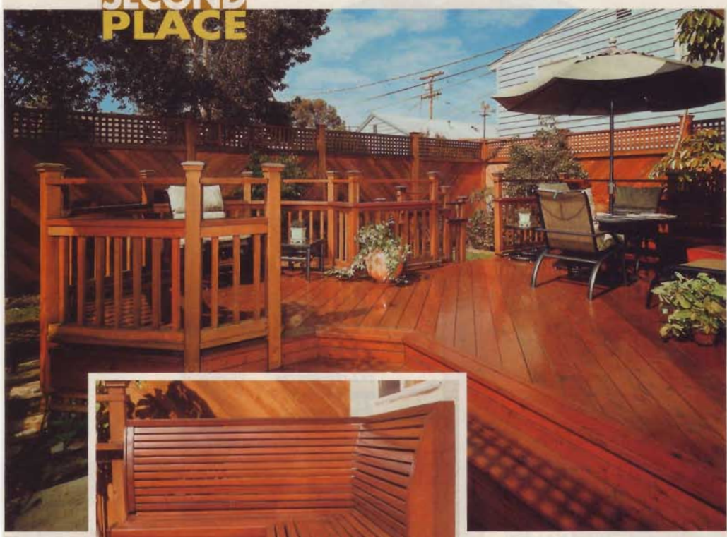
◀ Contoured Comfort Curved side rails and back supports create the form for the gently contoured seat slats, providing comfortable seating in this corner bench.
