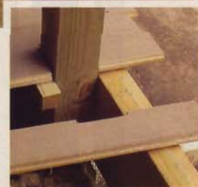
▲ A floor nailer (above) drives nails at an angle into the tongues of the flooring. A cleat attached to the post (right) supports notched boards.
