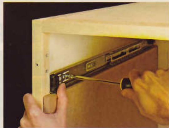
▲ Using a spacer to support the drawer slides makes installation easy and accurate.
