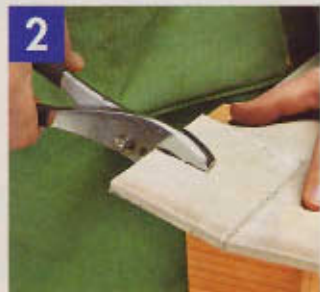
▲ Pliers provide leverage as you snap the waste piece free to form the notch.
