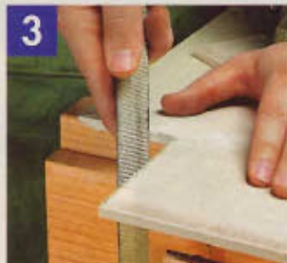
▲ A rasp makes quick work of smoothing the broken edge of the backerboard.
