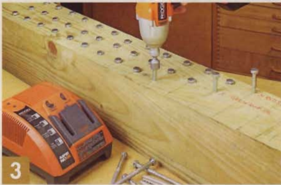
▲ Driving 5"-long lag screws into a 6x6, without pilot holes, gave us an excellent opportunity to see how long the batteries of these impact drivers would last.
