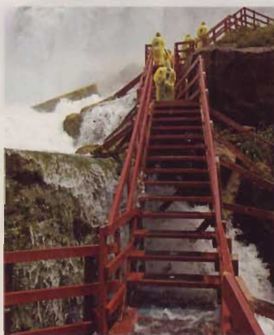
These decks don't get a break; they're deluged with water 24 hours a day.
