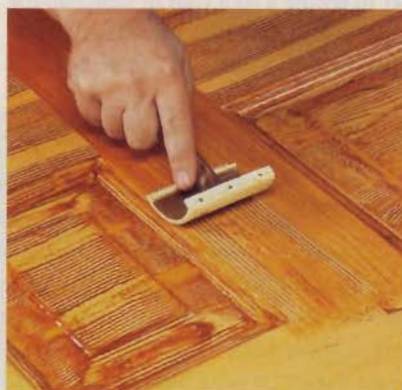
5] Make sure to follow the proper sequence as you grain the door to define the “joint lines.”
