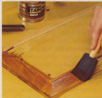
1] Working a section at a time, apply a thin coat of stain to the door. If your door has raised panels, stain those first.
