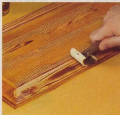
3] To grain the beveled edges of a raised panel, get an extra graining tool and trim it to fit the space.
