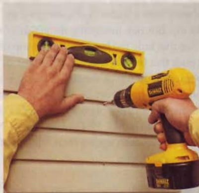
2] After pre-drilling mounting holes, move the panel into position, level it, and install it with 2" or longer screws.
