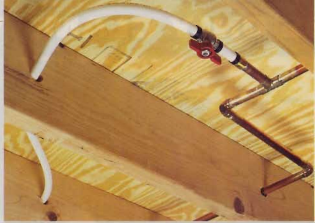
Flexible cross-linked polyethylene tubing, or "PEX," can be used in place of copper pipe for running hot- or cold-water lines. Check building codes to see if it's approved in your area.
