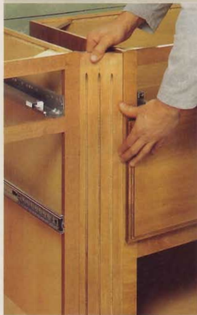
9] Slide the bump-out cabinet into place. Use the angled trim strips to fine-tune the fit.
