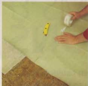
3] Roll out the rubberized underlayment, foil side down, and tape the seams.
