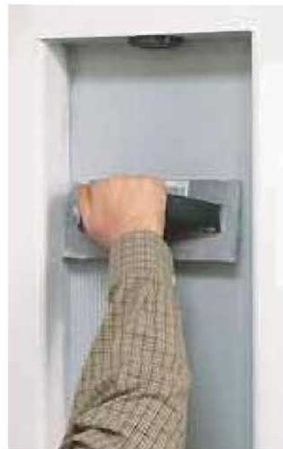
2] To adhere the tile, start by raking a thin bed of mortar across the back of the niche with a 1/8" notched trowel.
