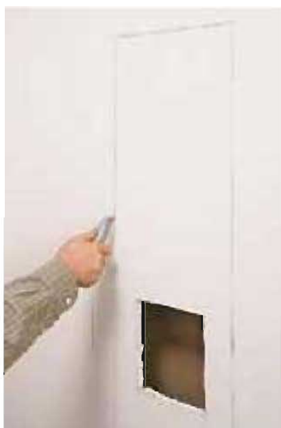
4] Use a utility knife to cut a clean, smooth opening. It will take a few passes to cut through the drywall.
