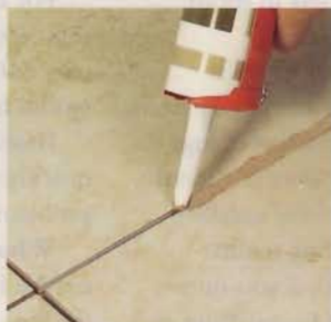
8] Apply Edge Flooring grout using a caulk gun or from pressurized cans.
