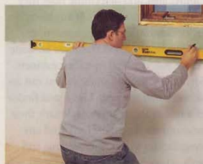
2] Draw the base cabinet level line on the wall, so you can align the top of the cabinets to this height.
