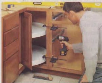
6] With the cabinets clamped securely together, drill pilot holes and then drive woodscrews through the face frames.
