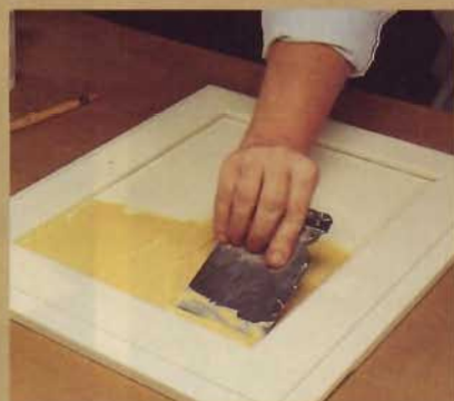
2] Use a putty knife to apply a thin ( \frac{1}{8} ") layer of Wood Icing. You can leave some of the ridges to add interest.
