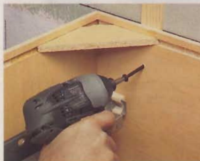
7] Now drive screws through the back of the cabinets at the shim locations to attach the cabinets to the wall.
