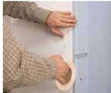
1] Cover the seam between the box and the wall with self-adhesive mesh drywall joint tape.
