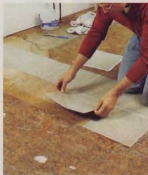
1] Self-adhesive vinyl tiles were a simple way to fill the footprints left by the old cabinets.
