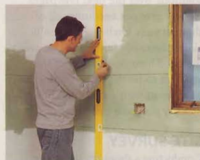
3] Outline each cabinet and any filler strips on the wall, so you'll have a quick reference as you're installing cabinets.
