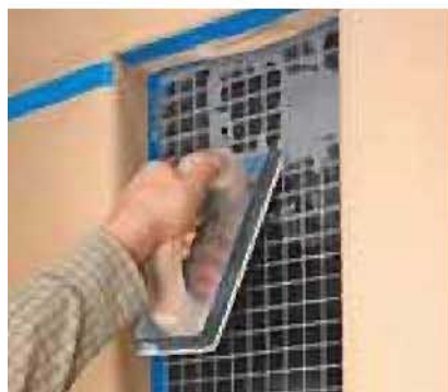
6] Mask the opening, and use a grout float to press grout between the tiles. Sponge off excess, then buff off any haze.
