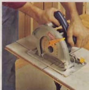
5] Cut tile using your circular saw or jig saw equipped with blades from Edge Flooring.
