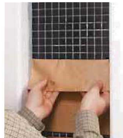
5] After 24 hours, sponge warm water over the paper facing, and carefully peel it off the tiles.
