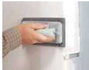
3] Let the compound dry for 24 hours, and then sand it smooth with a 220-grit sanding screen on a sanding block.
