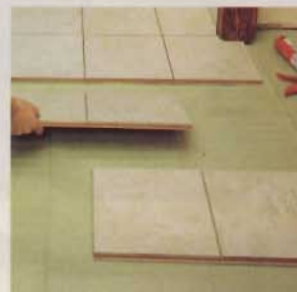
6] It's important to stagger the panels as you install them to avoid a continuous seam.
