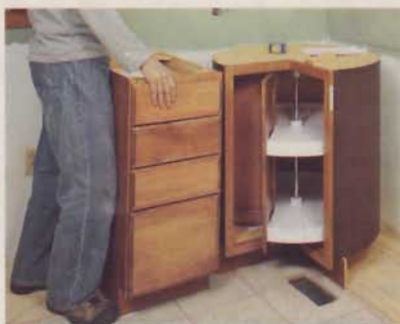
4] With the lazy Susan cabinet in place, we moved the adjoining cabinets into position to “capture” the corner unit.
