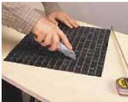
1] To cut a sheet of tile to size, flip it upside down, and use a utility knife to slice through the paper facing.
