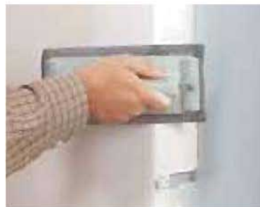
4] Now use the sanding block to smooth the rounded corners. Then apply another coat of joint compound.
