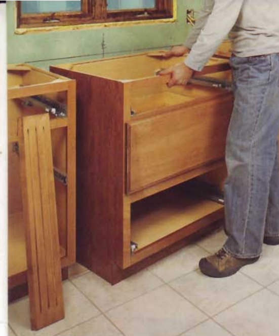
9] Slide the bump-out cabinet into place. Use the angled trim strips to fine-tune the fit.
