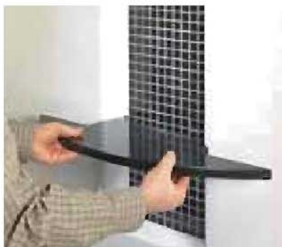
7] When the grout dries, check the fit of the shelf. Sand or file the back edges as needed to produce a tight fit.
