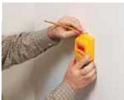
1] To determine the location of the studs, sweep a stud finder across the wall, and mark their positions.
