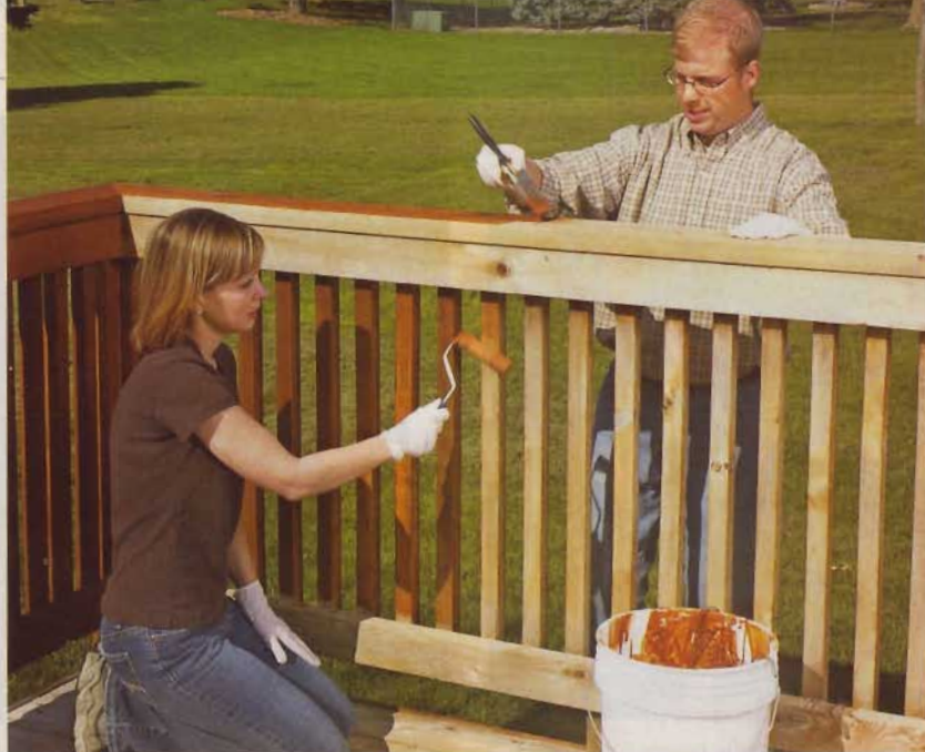
4] Stain the deck rails and balusters first. Use a small roller to coat most of the surfaces and a synthetic bristle brush to fill any areas where the roller can't reach. Also use the brush to smooth the stain with the grain direction.
