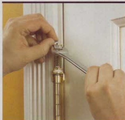
A nut and locking pin allow you to adjust the force of a hinge-pin closer.
