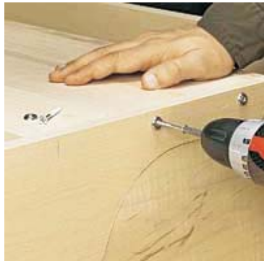
FIGURE 4 With both pivoting arms in place, you can now attach the work surface between them using 2" Fh Woodscrews and finish washers.
