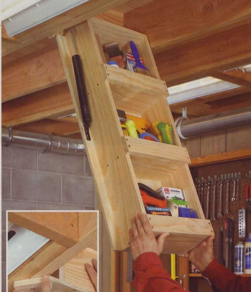
This storage bin takes advantage of the last unused space in the shop—the space between the exposed floor joists. A wood turnbutton (left) "locks" the bin in place.
