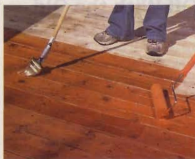
5] The most efficient way to finish the deck boards is as a two-person team, with one person applying the stain with a roller and the second person smoothing the stain with a brush. Attach a brush to an extension handle with duct tape to save your back.
