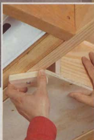
This storage bin takes advantage of the last unused space in the shop—the space between the exposed floor joists. A wood turnbutton (left) "locks" the bin in place.
