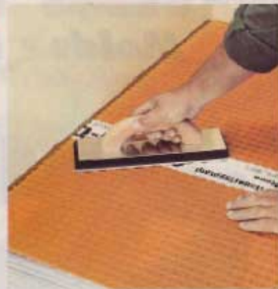
3] Press the Ditra using a sponge float to solidly embed the fleece layer into the thinset mortar.
