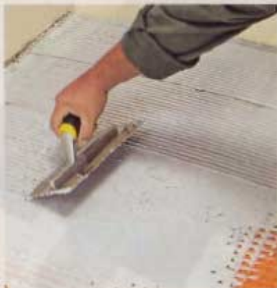
5] Now use a \frac{1}{4} " x \frac{1}{4} " notched trowel to apply the "bonding" layer of unmodified mortar directly over the scratch coat.
