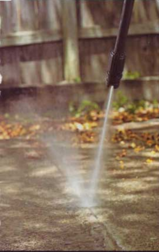
A focused stream can clean dirt and weeds out of concrete seams.
