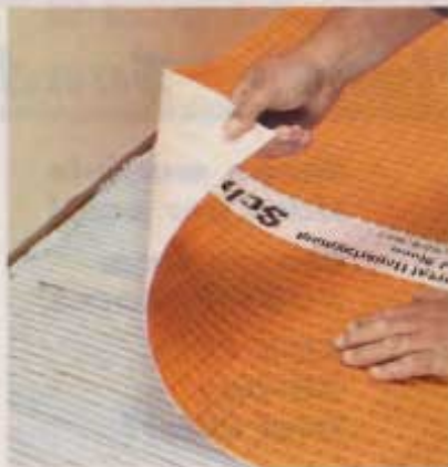
2] Roll Ditra onto the mortar with the fleece side down. Simply butt pieces of Ditra together to cover the entire floor.
