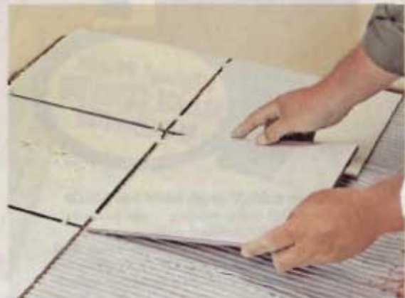
6] Install the floor tile as usual, using spacers to ensure uniform alignment. Be sure to set the tiles firmly in the mortar.
