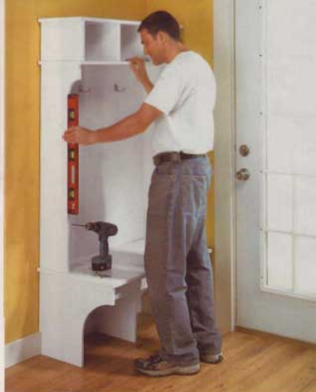
5] Make sure the locker assembly sits level from front to back and side to side. Then screw it to the wall studs.
