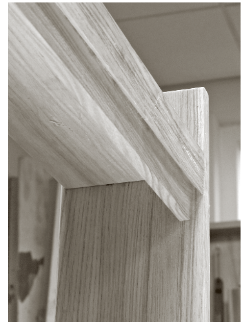
A hidden French cleat slips over a matching angled cleat to hold the shelf to the wall.
