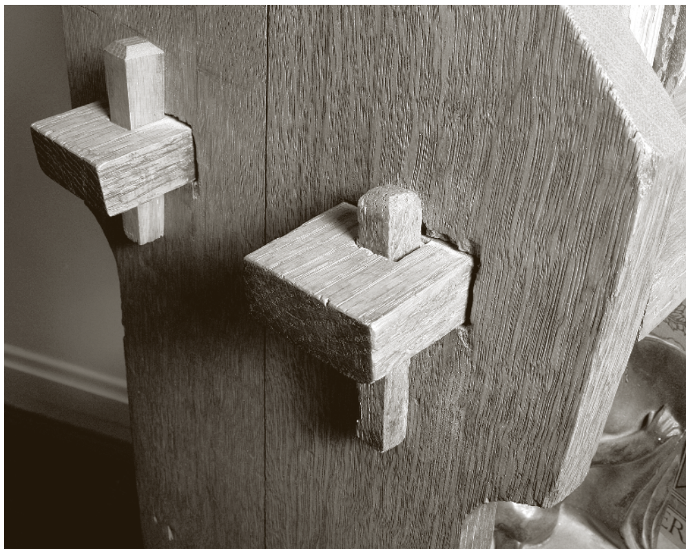
The torn grain, gaps and general loose fit around these through-mortises are unacceptable to the modern woodworker – though these defects were once common. This is an Arts & Crafts bookcase that once graced a church library in Lexington, Ky.
