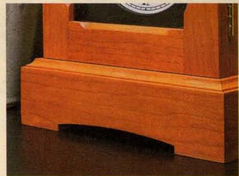
▲ The front base trim of the mantel clock features a stopped arc that terminates in a shoulder at each end.
