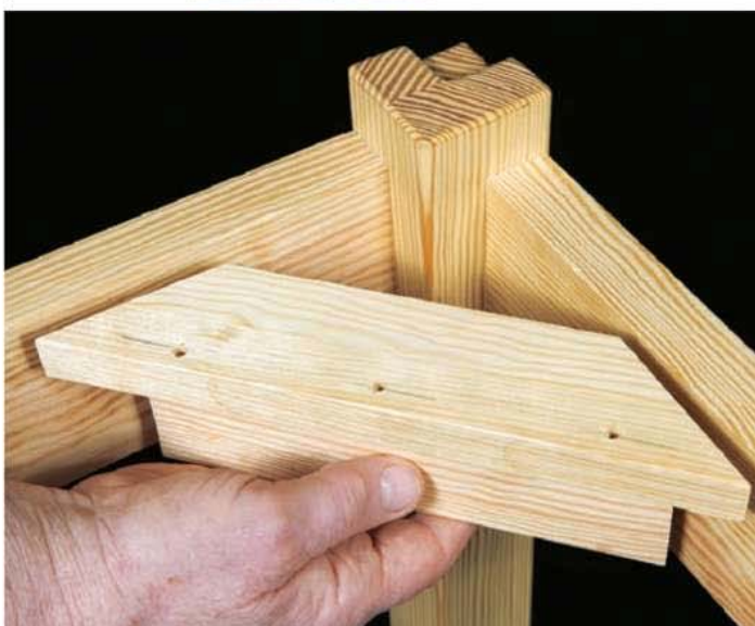
The angle-shaped corner block (above) serves two purposes. It adds a great deal of resistance to stress on the joints, and screws driven through its oversized holes hold the top in place.
