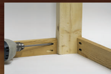
Assemble flush & corner joints
