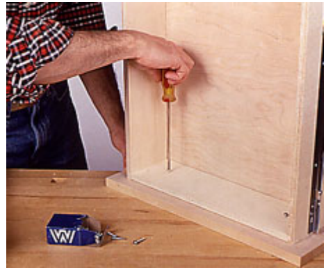
21--Attach the drawer faces to the drawer
