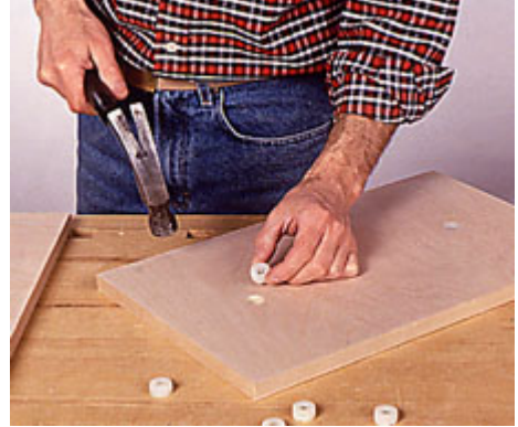
20--Bore holes in the back side of each drawer face for the adjusters. Then, tap adjusters into the holes. No glue needed.
