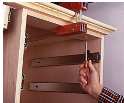
19--Place top on the desk pedestals and clamp in place. Bore pilot holes through the rails into the top and install screws.
