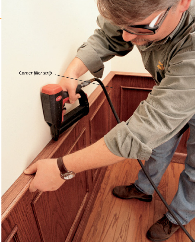
With the stud locations marked ( top left ), nail the base support and hanging strips in place. Next, attach the assembled panels to the hanging strips with the panels resting on the base support strip ( bottom left ). Next, miter the baseboard and cap mouldings in the corner and nail them to the panels ( top ). Note the 3" filler strip necessary to complete the corner.
