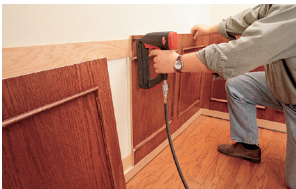
With the stud locations marked ( top left ), nail the base support and hanging strips in place. Next, attach the assembled panels to the hanging strips with the panels resting on the base support strip ( bottom left ). Next, miter the baseboard and cap mouldings in the corner and nail them to the panels ( top ). Note the 3" filler strip necessary to complete the corner.
