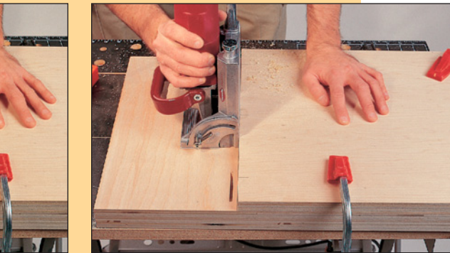
Now turn the biscuit joiner on its head and cut the slots in the panel. Use the layout lines on the partition and the centerline on the bottom of the tool to properly line up the biscuit joiner.
