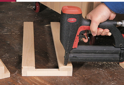
I used my brad nailer to tack the channel bottom in place between the two channels through the front and through the sides. Be careful about shooting too close to the end of a piece to avoid blow-outs.
