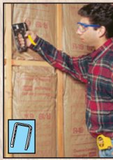
Install Insulation
