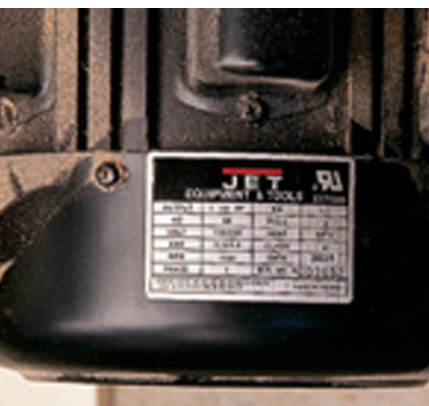
This nameplate is on our band saw's motor. Note that at 115V, this motor draws 11.5 amps. At 230V, it draws half the amps: 5.8.
