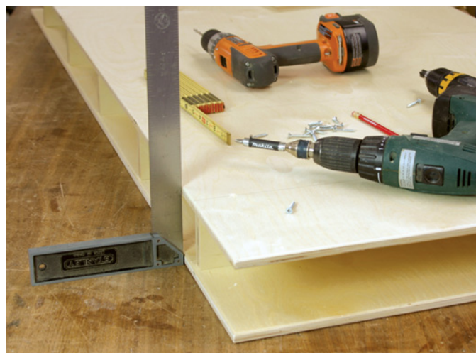
With the ribs attached, the bottom is simply screwed in place. Countersink the clearance holes, and use a square to help align the top and bottom pieces before sinking the first screw.
