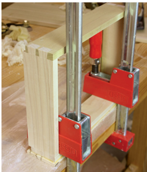
Build the drawers with through-dovetails. Then glue a piece of 1/4"-thick veneer to the front.
