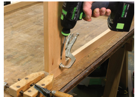
The face frame is put together with pocket screws before being glued in place on the assembled cabinet box. Two clamps hold the stile on edge so that I can see and reach both sides of the joint.
