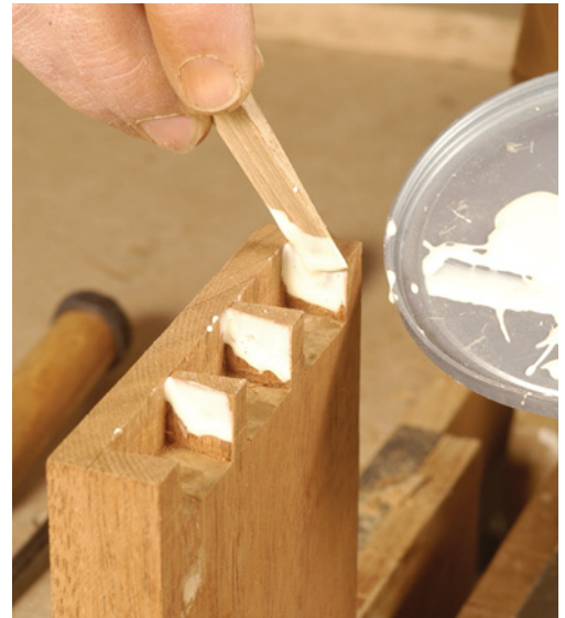
First test the joint by just starting the two pieces together. Pare away any material that would seem to interfere with the joint. Then apply a bit of glue to the sides of the pins and assemble the joint.
