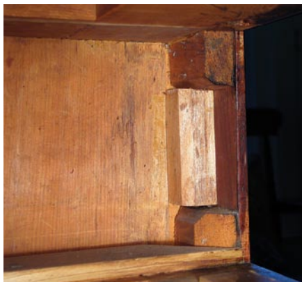
Glue-block strength. These glue blocks in the inside corner of a mid-19th-century Empire chest-of-drawers are still strong. Glue blocks were commonly used in corners to add strength.
