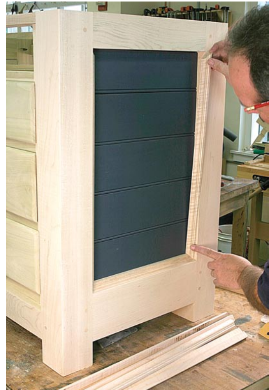
Picture-frame moulding. The panels on the base are held in place by the moulding that is installed in picture-frame fashion – the corners are mitered.
