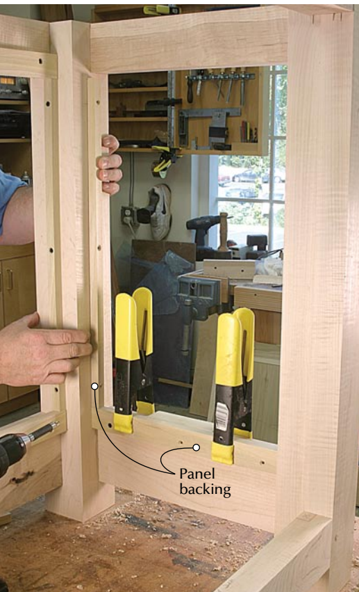
Sandwiching the panels. The panel backing, along with mouldings, hold the panels in position. The backings are screwed to the inside face of the rails as well as to the legs.
