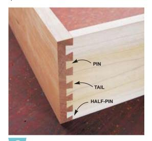
Half-blind dovetails make an incredibly strong joint. They're particularly suited for drawers: you can't pull dovetails apart by yanking on a drawer front. Half-blind dovetails are only visible from one side of a corner: you can't see them from the front (that's why they're called "half-blind").
